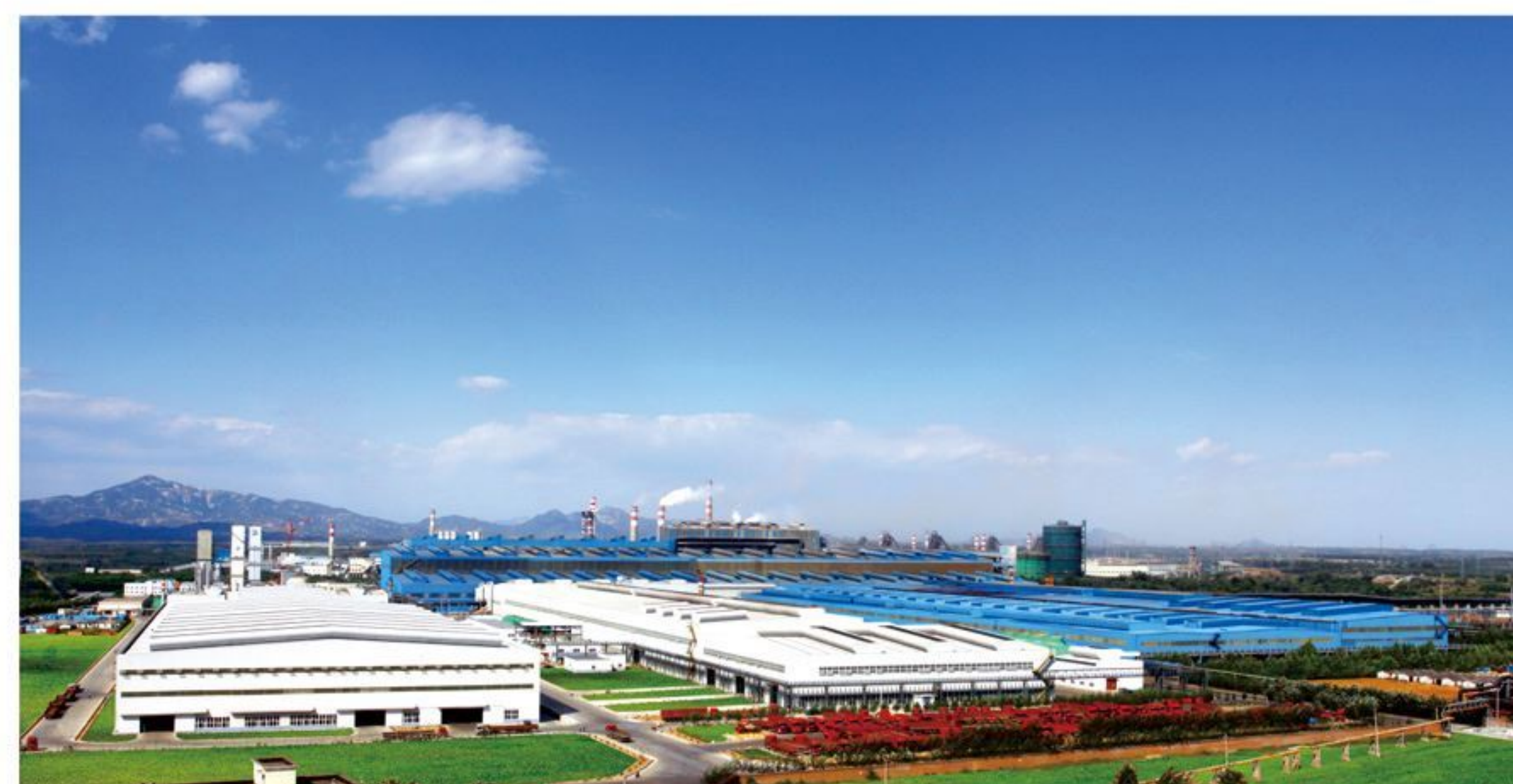
Hebei Jingye Steel Co., Ltd. 230m 2 sintering flue gas denitrification project
