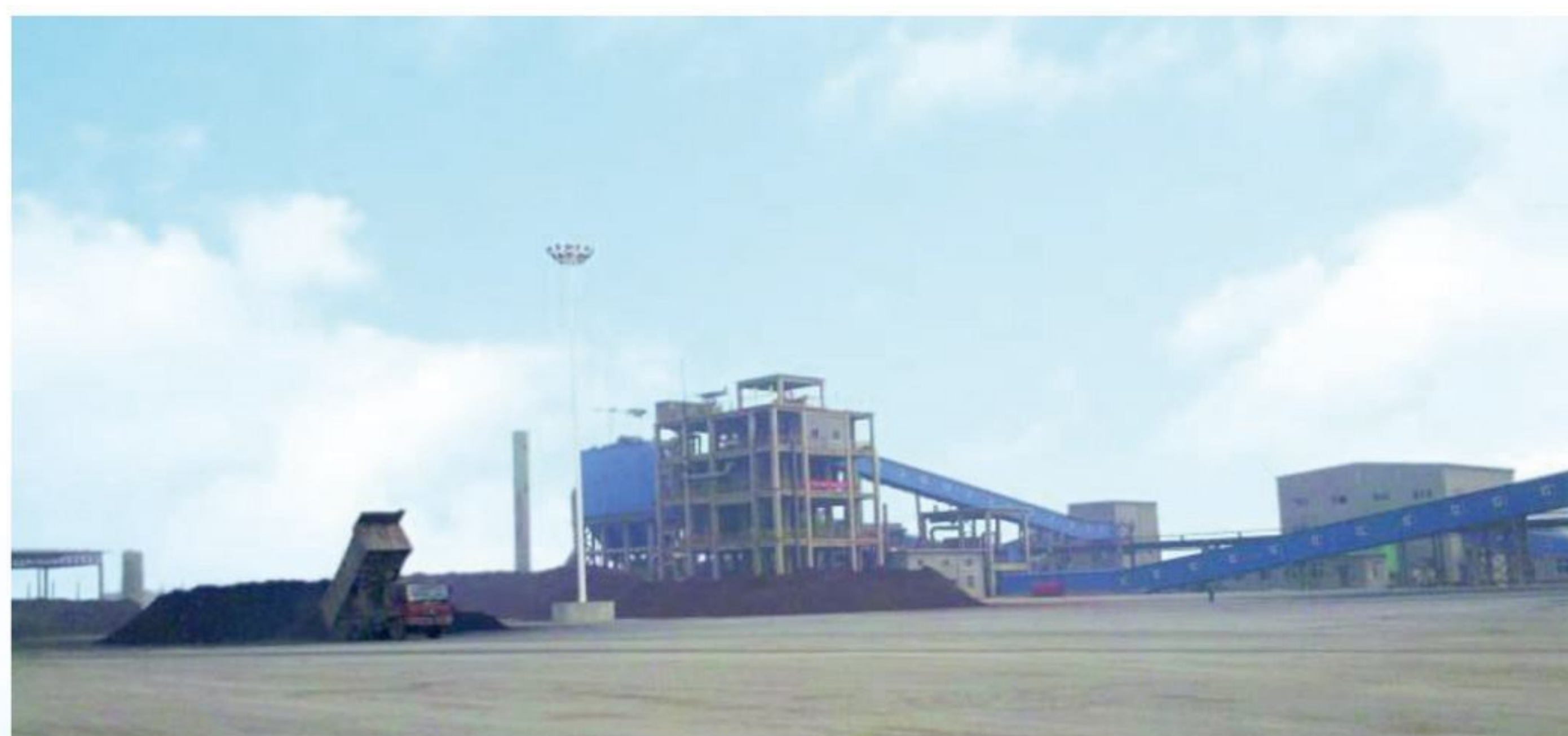
Shanxi Zhongsheng Steel Co., Ltd. 180m 2 sintering flue gas denitrification project
