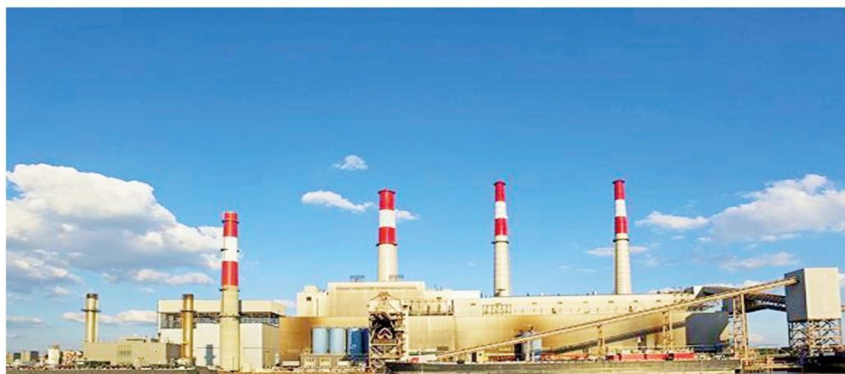
Hebei Anfeng Steel Co., Ltd. 2*180m 2 +360m 2 sintering flue gas denitrification project
