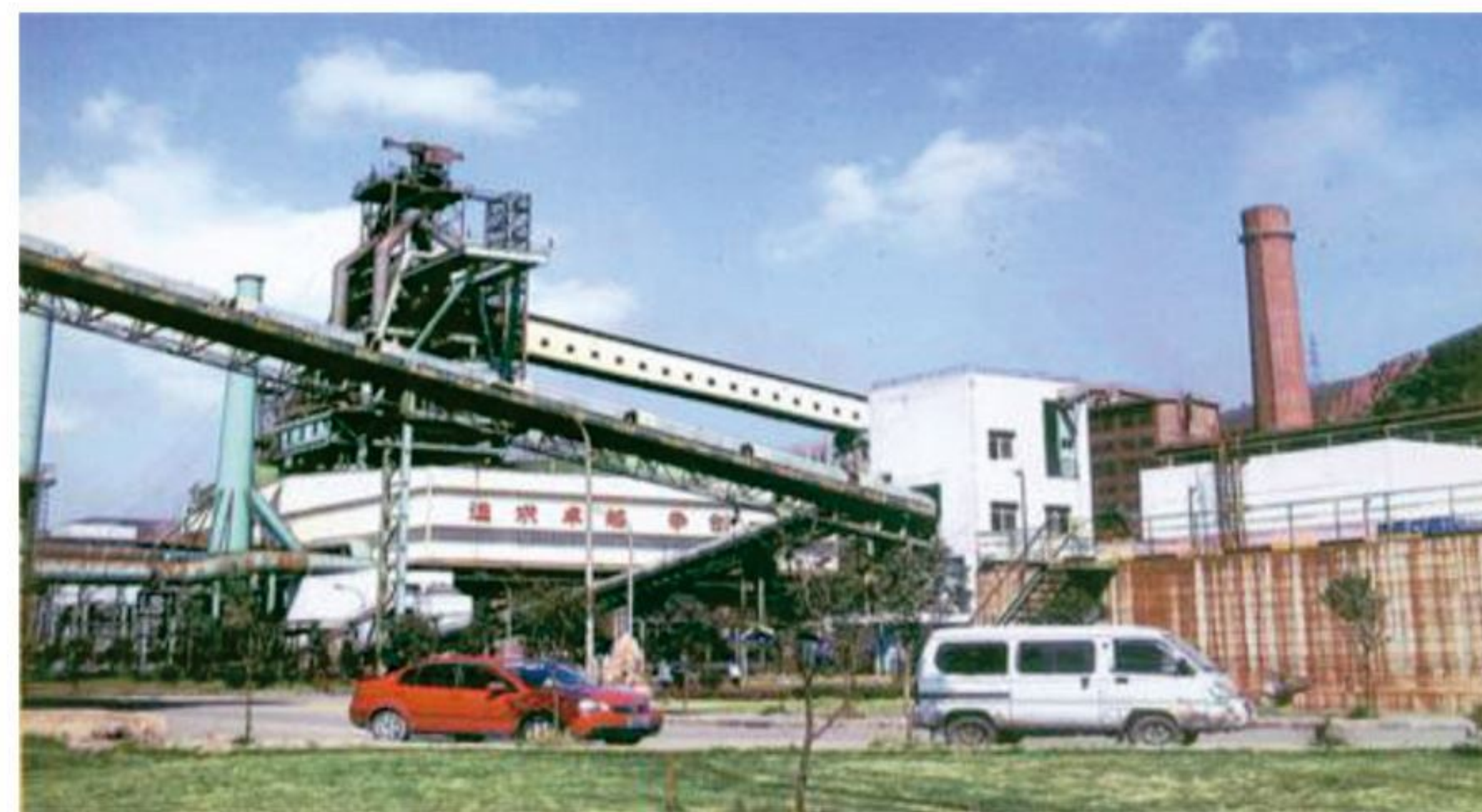
Wu'an Yuhua Iron and Steel Co., Ltd. 2*200m 2 sintering project
