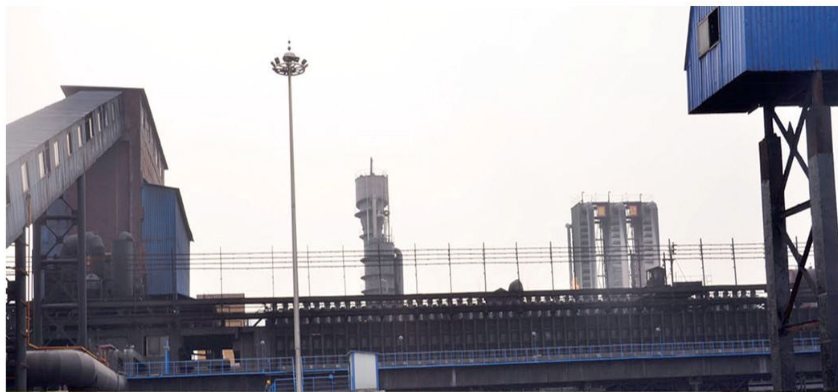
Fengfeng Mining Area Hexin Iron and Steel Co., Ltd. 120m 2 sintering catalyst project
