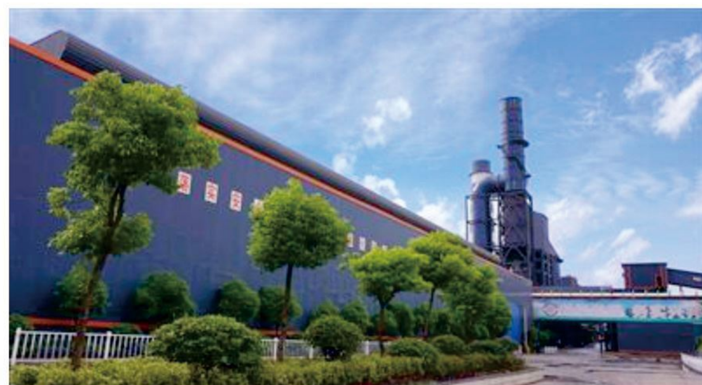
Danyang Longjiang Iron and Steel Co., Ltd. 70+130m 2 sintering flue gas denitrification project
